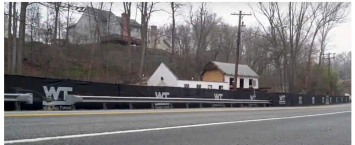
Ongoing church construction post-storm from the side of Seven Locks Road.
