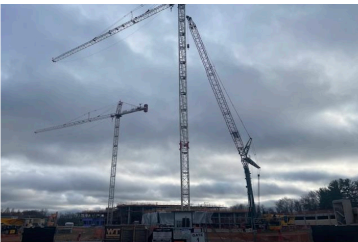
Grandview site with large cranes.
