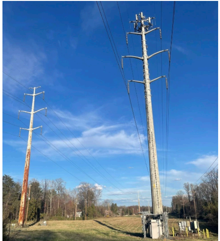
Two towers; one significantly rusted.
